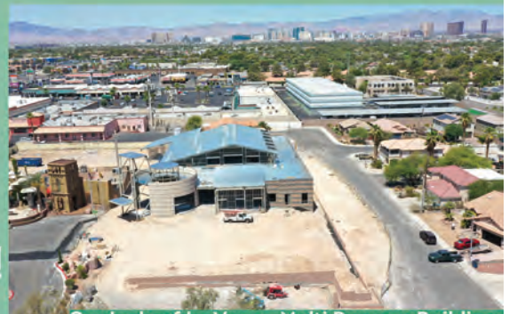
Our Lady of La Vang - Multi Purpose Building
