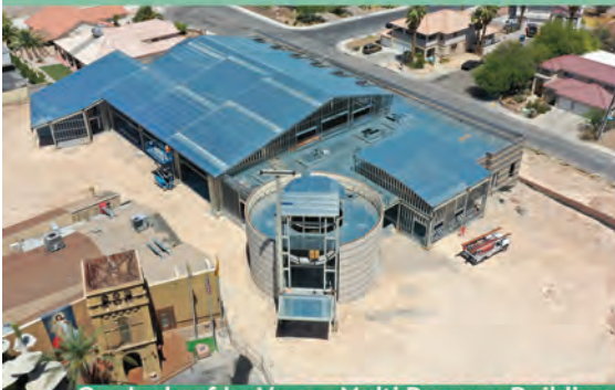
Our Lady of La Vang - Multi Purpose Building
